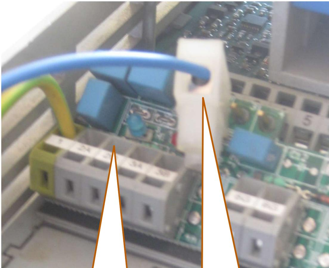
**Remove wire from LP pressure transducer at terminal 2B**
